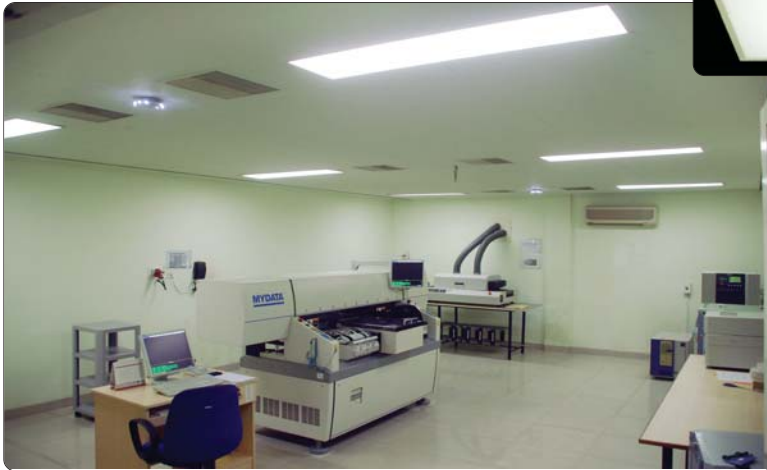
Room Size: 20 X 28 feet Indirect T8 Fluorescent Luminaires 6 X 72W = 432W with an Average Illumination of 150 LUX Replaced with 6nos 1' X 4' 24W Troffer Lights 6 X 24W = 144W Obtaining Average Illumination of 150 LUX
