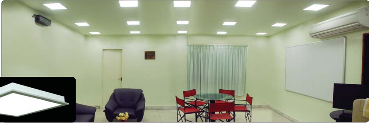
Room Size: 18 X 20 feet, Indirect T8 Fluorescent Luminaires 5 X 72W = 360W with an Average Illumination of 125 LUX Replaced with 25nos 1'x1' 6W Troffer Lights 25 X 6W = 150W Obtaining Average Illumination of 180 LUX
