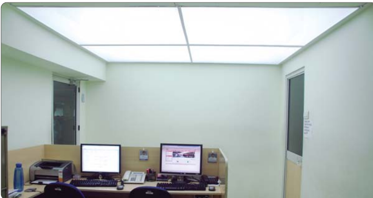
Room Size: 8 X 8 feet, Indirect T8 Fluorescent Luminaires 2 X 72W = 144W Replaced with Sky Light @ 1Watt / sqft = 64Watt. Average Illumination of 200 LUX
