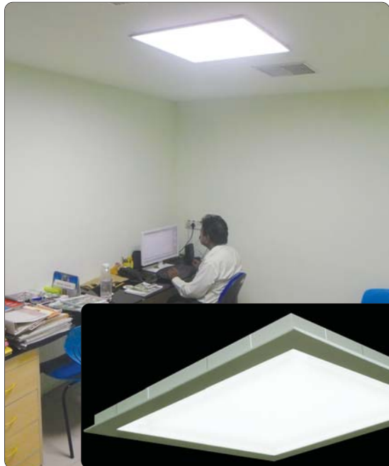
Room Size: 10 X 10 feet Indirect 2' X 2' CFL Luminaires 2 X 36W = 72W with an Average Illumination of 100 LUX Replaced with 2' X 2' 40W Troffer Light Obtaining Average Illumination of 200 LUX
